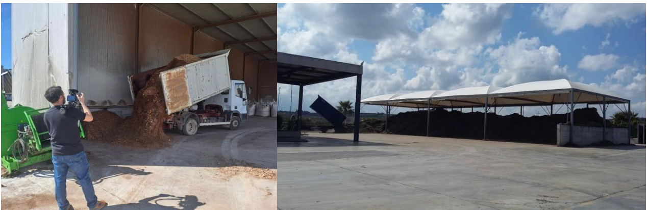
Figure 5 - Storage area at the plant
