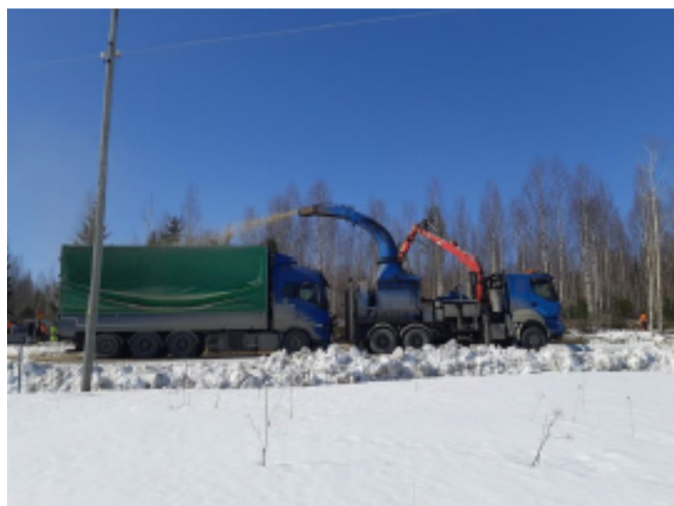
Figure 6. Chipping at the roadside directly to the chip-truck.
