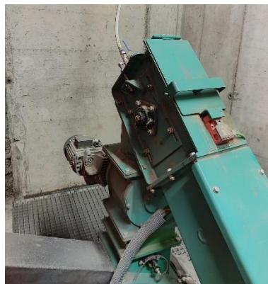
Figure 11. Additional cutting system.
