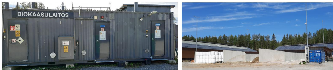
Figure 6. Biogas plant (left) and grass silos (right). Photos: Saija Rasi.
