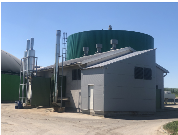
Figure 2. Cogeneration block at Biogal. Source: BIOGAL.
