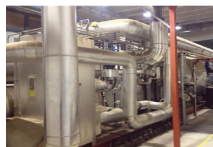
FIGURE 7. The 1MW ORC turbine
