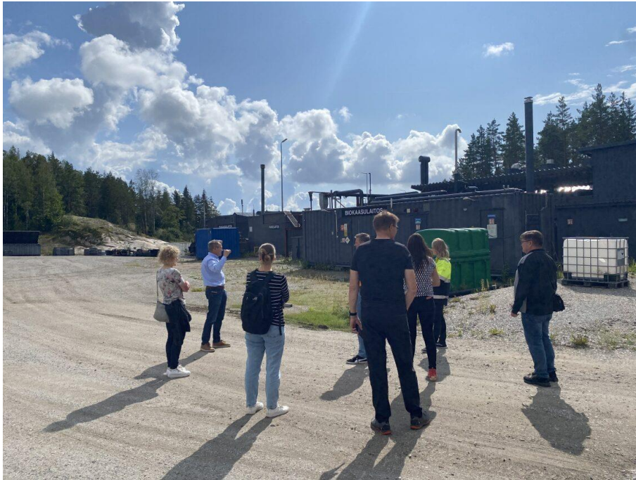
Picture: Visiting the experimental biogas plant. The plant utilizes cow manure and grass as a feedstock.
