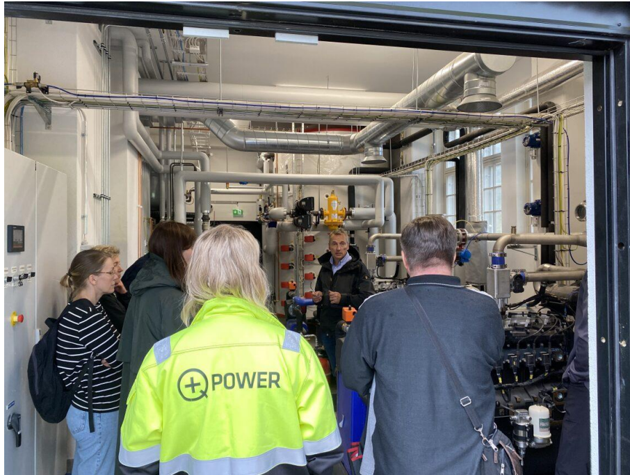
Picture: CHP units are used to generate heat and electricity for the premises located at the farm.
