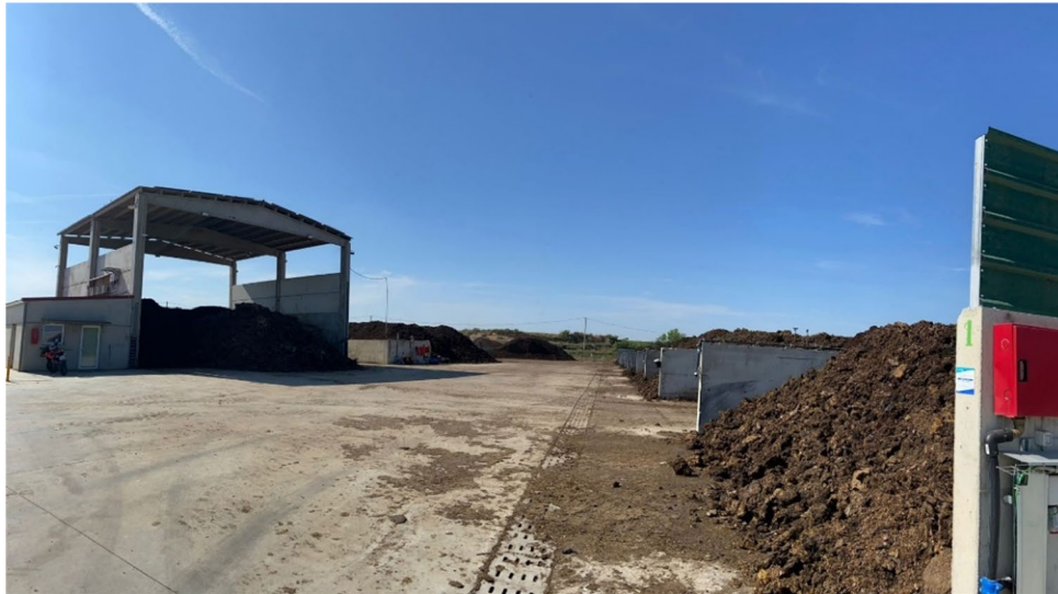
Figure 3. Biomass storage site
