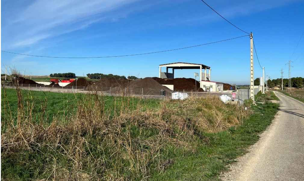
Figure 2. Alcarràs composting plant
