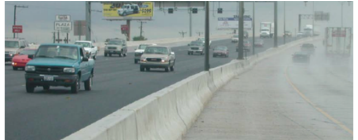
The difference between a conventional asphalt and rubberized asphalt without spray water
