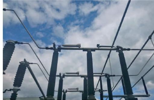
**FIXED CONTACT:** LC 259 silvered fixed contact blade and complete of fixing screws and stainless steel pressure groups.
