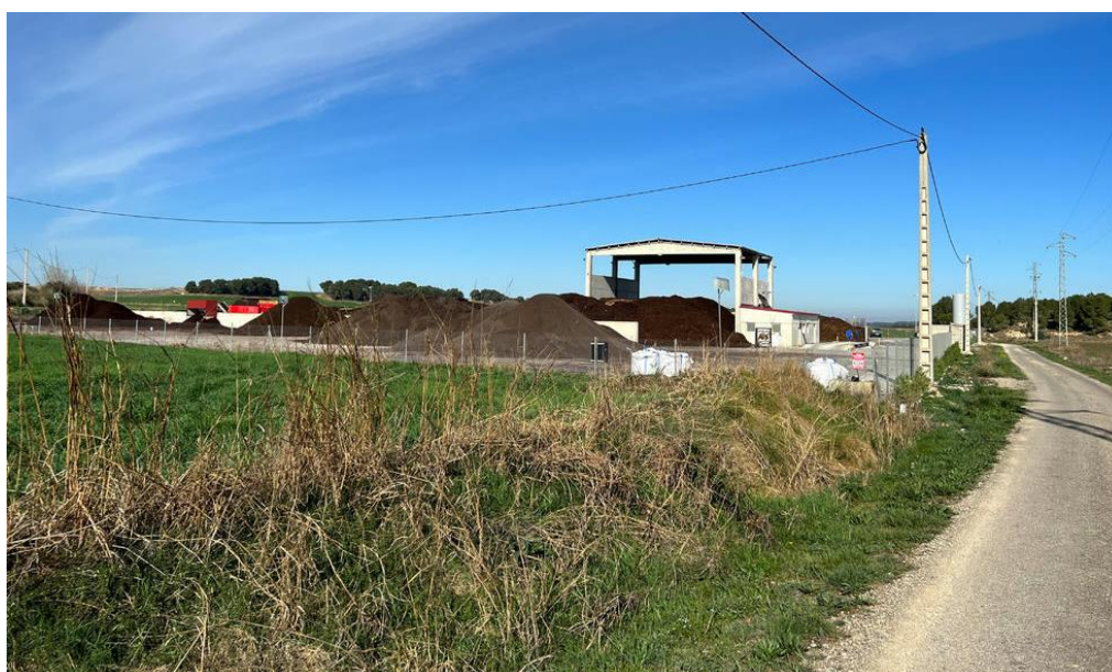
Figure 2. Alcarràs composting plant
