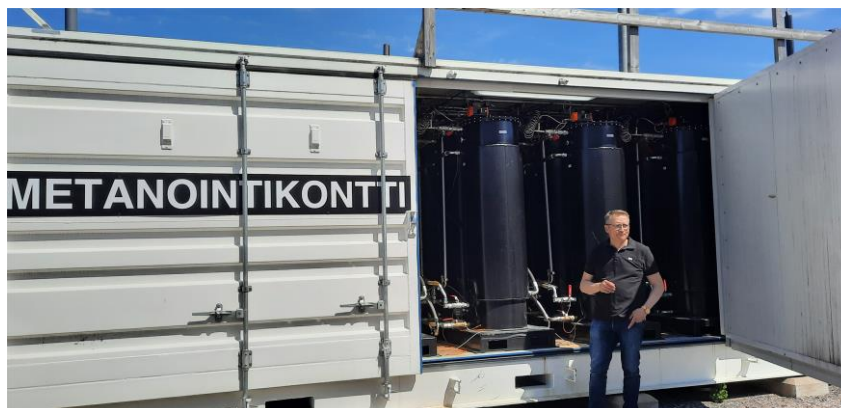
Figure 7. Biological methanation unit at Qvidja farm. Photo: Saija Rasi.
