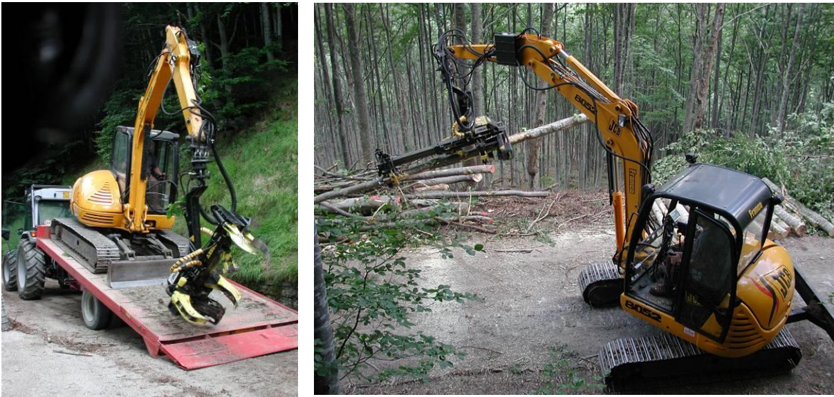
Figure 4 – The light stroke processor used by Santini Timber. The processor is installed on a mini-excavator and the whole machine is compact and light enough for easy relocation and trouble-free maneuvering even in constrained-space work sites. The machine is also cheap and reliable. It is now 10-years old, and it still runs smoothly. Professional handling and careful maintenance is all it takes to guarantee a long service life.
