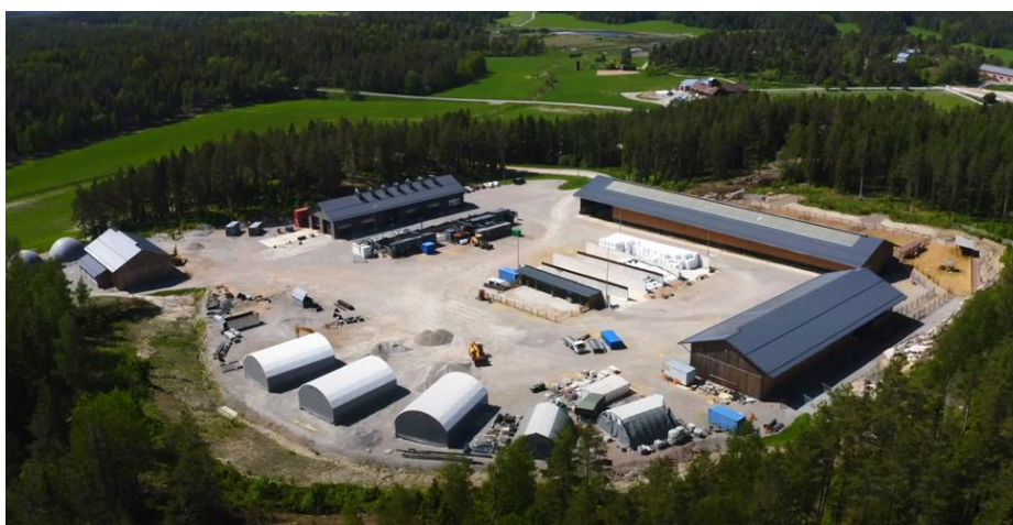
Figure 4: Qvidja farm provides a research and development environment for various renewable energy technologies. Video: “The farmer is the solution”
