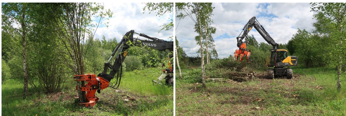
Figure 1. Felling trees, bushes using a Westtech Woodcracker hydraulic shear head
