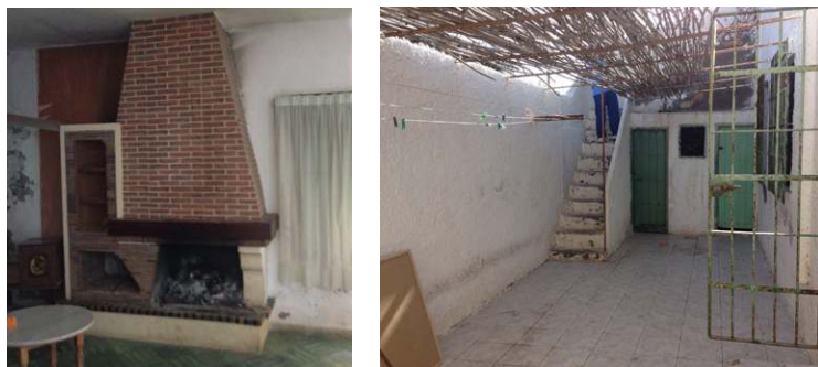
En la Ortilla - Prima, Ante Operam, Before renovation
