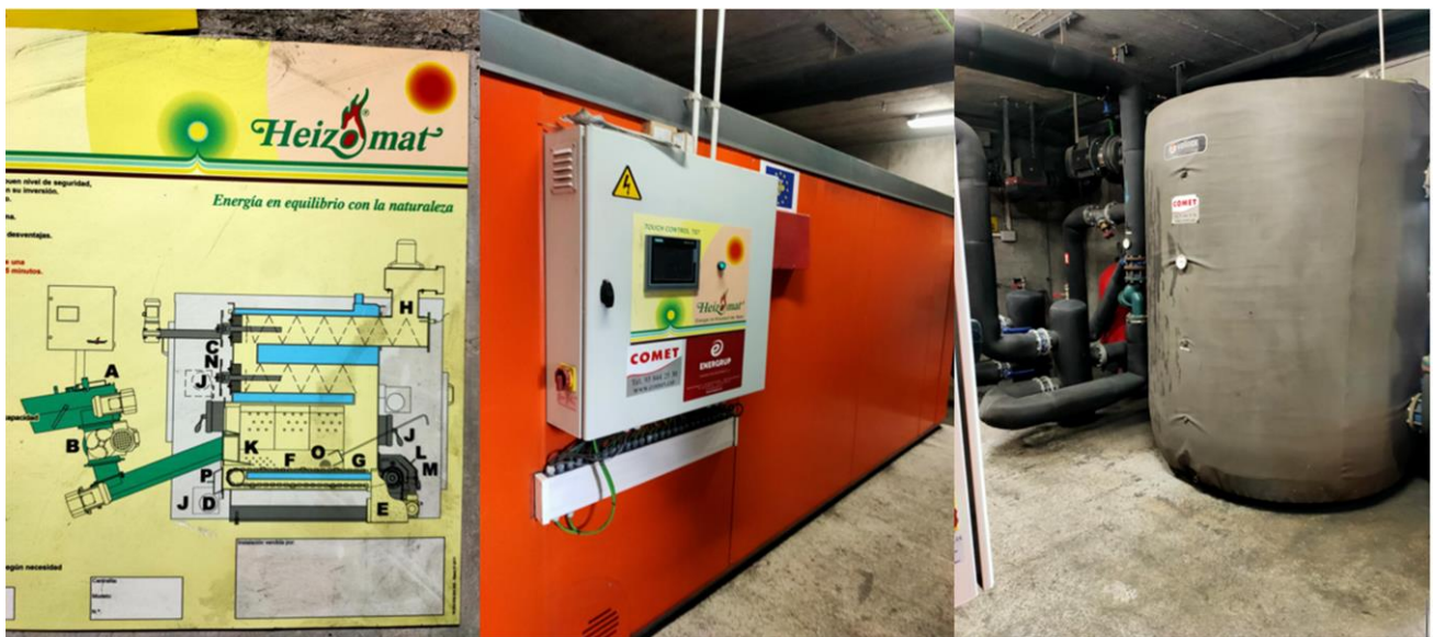
Figure 10. Boiler and district heating system.
